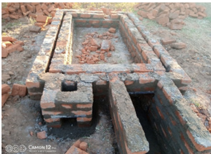
Fig.25: Construction of Adam Retort Kiln in Kitui Energy Centre
