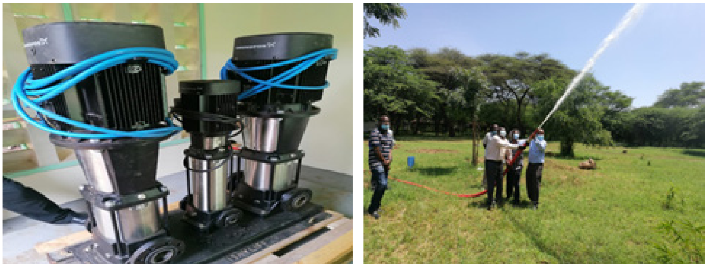
Fig.32: Fire pumps and commissioning of the completed works
